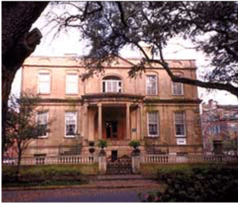
The stucco on the early-19th century Richardson-Owens-Thomas House in Savannah, Georgia, is a type of natural cement.
