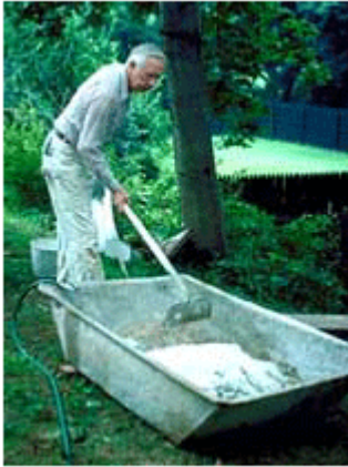
The dry materials must be mixed thoroughly before adding water to make the stucco.
