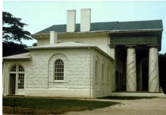
The stucco finish on Arlington House, Arlington, Virginia, was marbled in the 1
