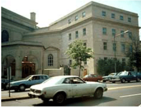
The new addition on the right is stucco scored to imitate the limestone of the historic building on the left.
